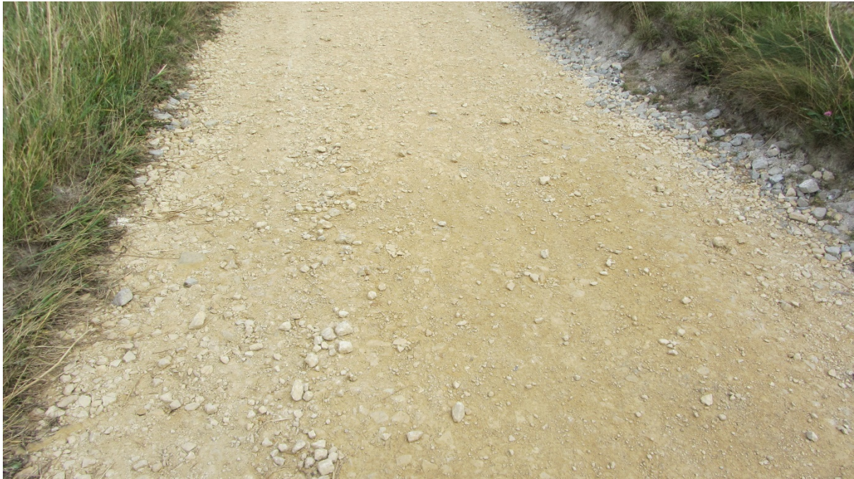
The finished surface of limestone and finings
